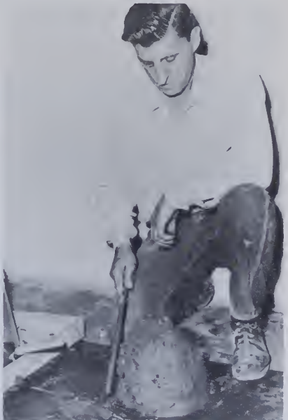
Tapping the concrete to observe the plasticity
